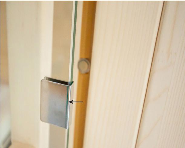
Fig. 35: Assembly of sleeve plate
