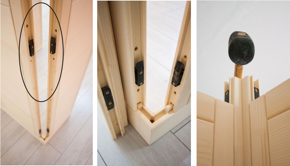
Fig. 4: Connecting wall elements with corner post
